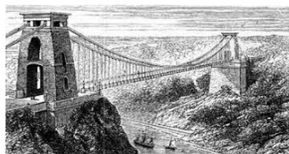
Clifton Suspension Bridge, Bristol
